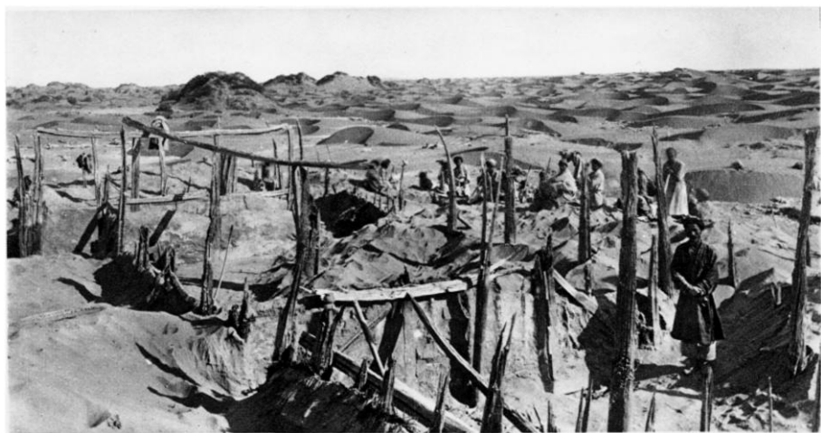
33. CENTRAL HALL AND OFFICE ROOM IN RUINED RESIDENCE, N.XXIV., ANCIENT SITE BEYOND NIYA RIVER END, AFTER EXCAVATION
